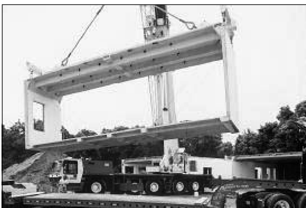
Fig 4. On-site assembly of prefabricated panels
