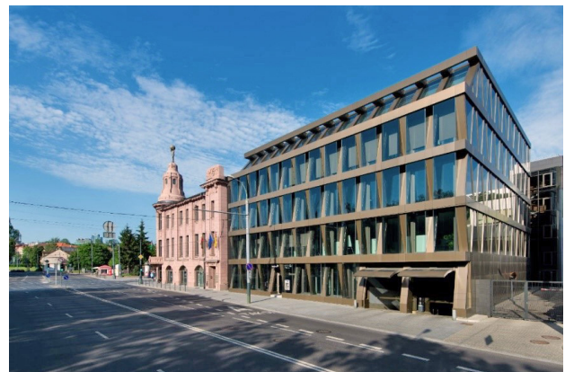
1 paveikslas. Tiriamasis pastatas, Gedimino pr. 35, Vilnius Figure 1. Building of a case study, located at Gedimino ave. 35, Vilnius
