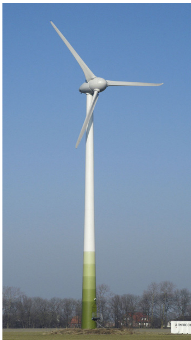
Fig. 2. Investigated wind turbine in Vydmantai
