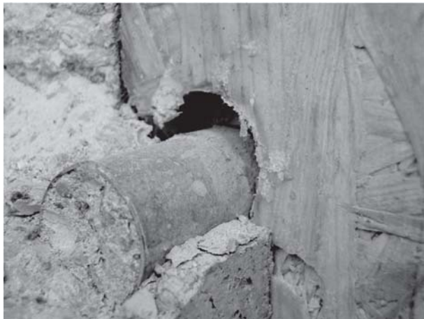
Fig 8. View of failure in specimen connection
