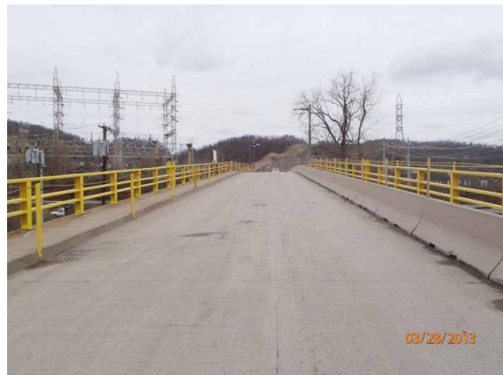
Figure 6. Access road bridge deck at Cardinal plant
