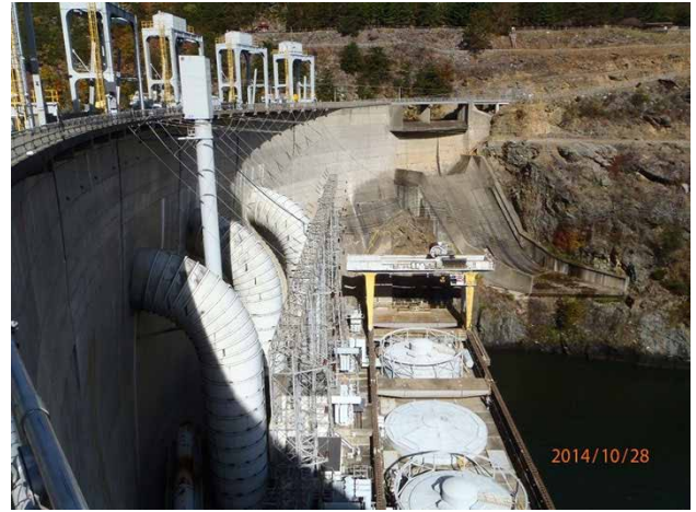
Figure 9. Smith Mountain Hydroelectric facility and dam
