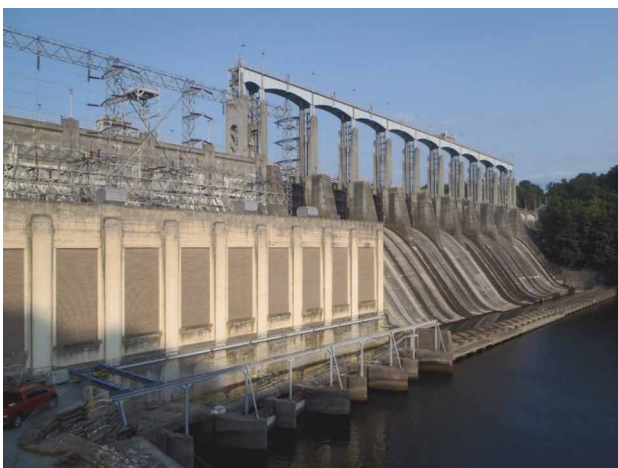
Figure 4. Claytor Hydroelectric facility and dam
