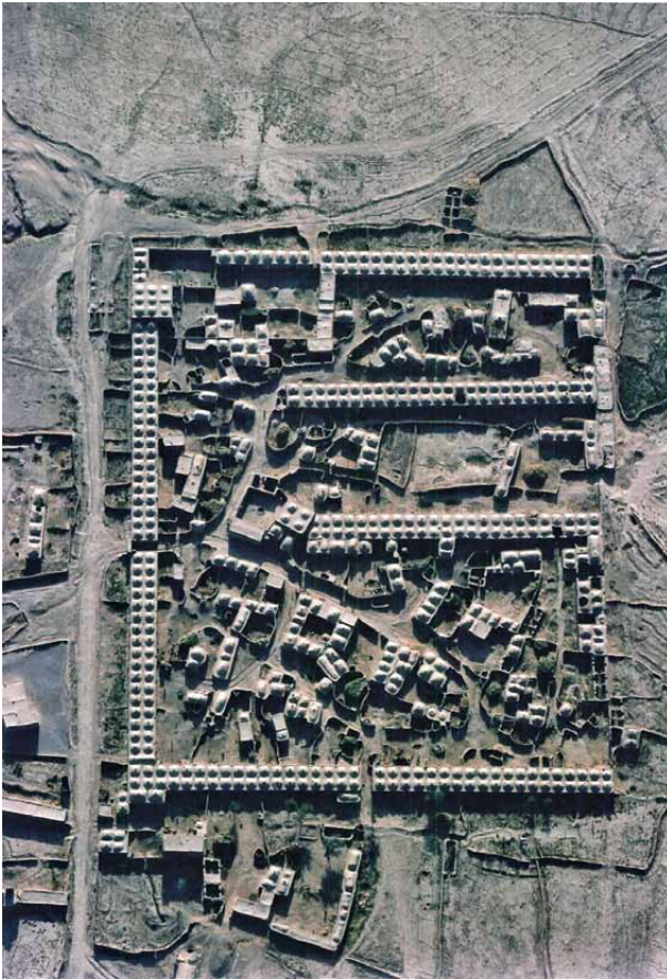
Fig. 10. Inhabitable walls. Aerial photo of a small city in Khorasan, Iran. Source: Gerster, G. 2008. Paradise Lost: Persia from Above . London: Phaidon.
