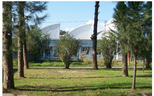
Figure 7. Manufacturing hall (photo is taken by the author in 2023)
