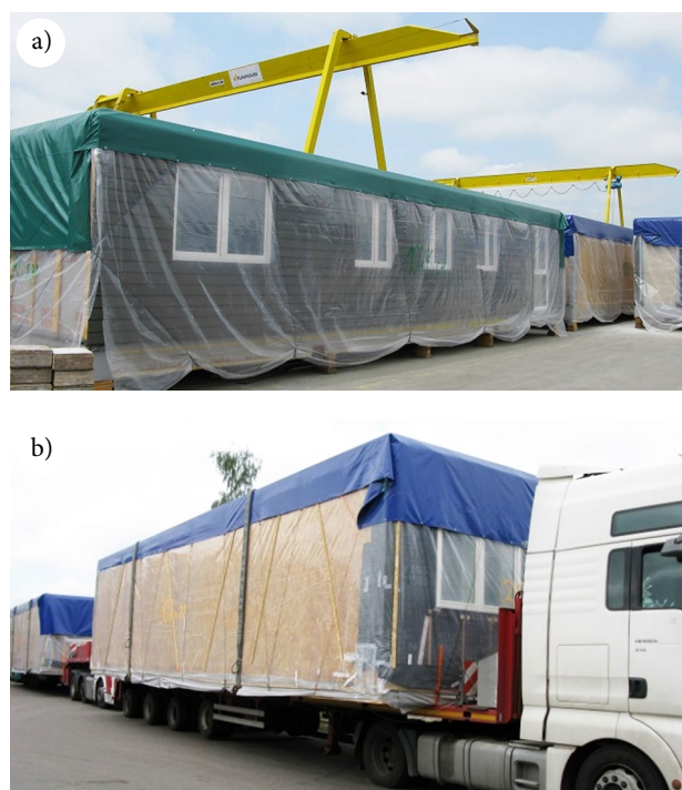
Fig. 9. Loading and transportation to the site
